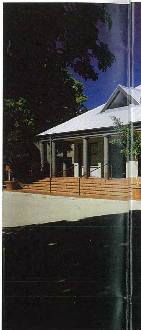
Entrance, New Farm Clinic, Brisbane This is a proposed asset of the Company
