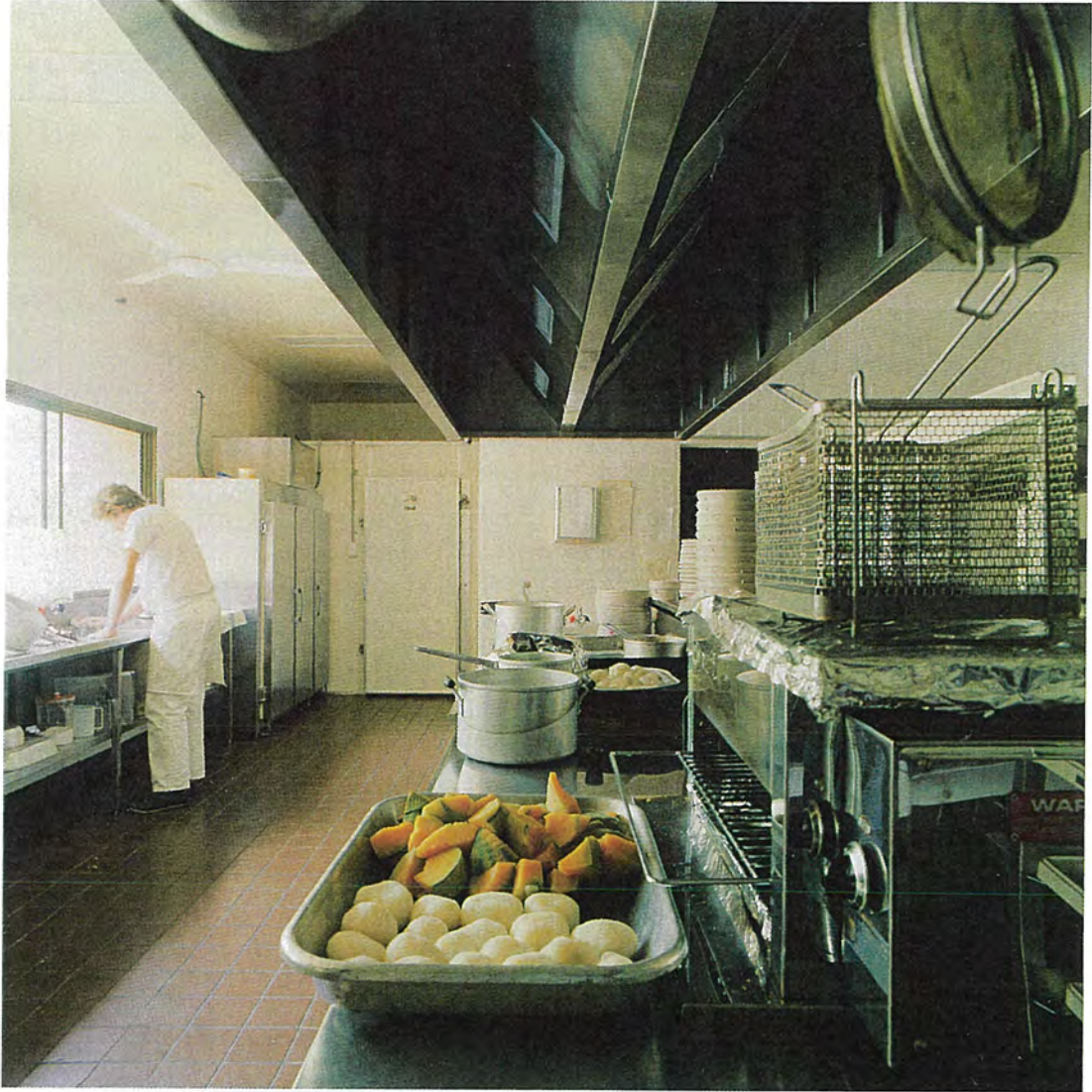
Part of the kitchen of Baringa Private Hospital, Coffs Harbour, New South Wales This is a proposed asset of the Company
