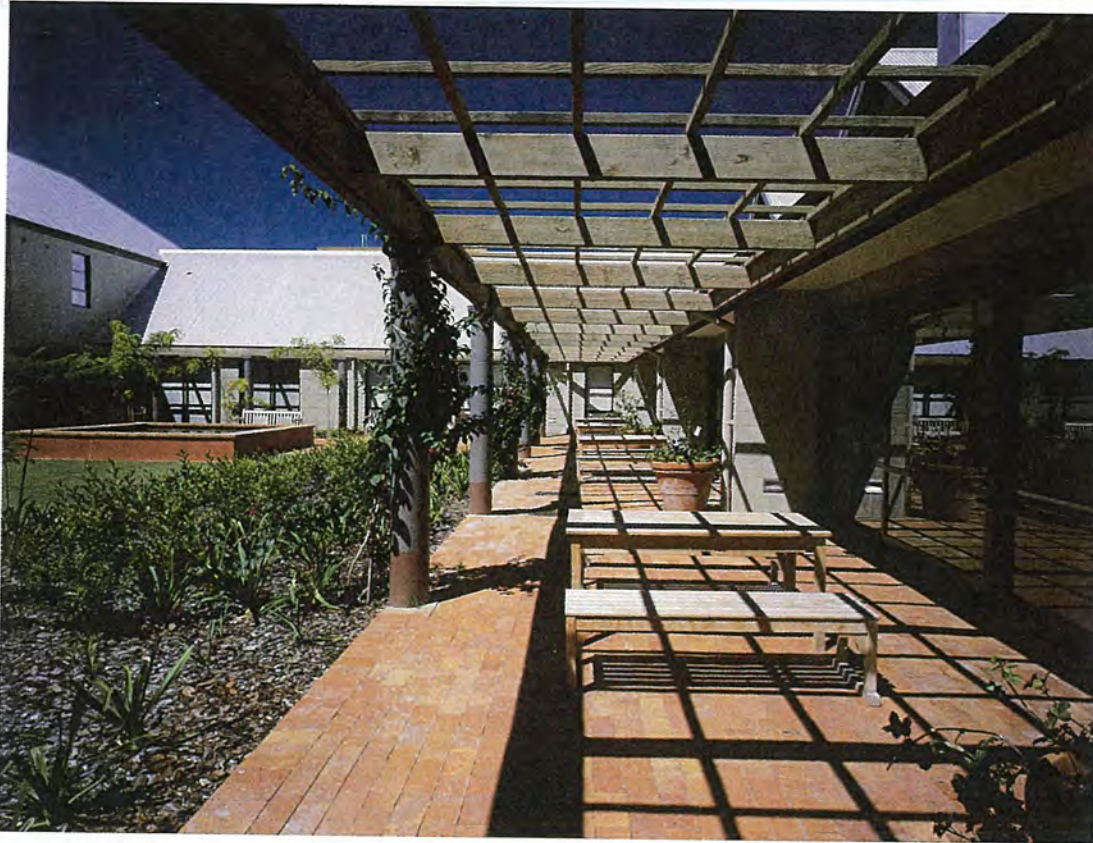
Courtyard, New Farm Clinic, Brisbane This is a proposed asset of the Company
